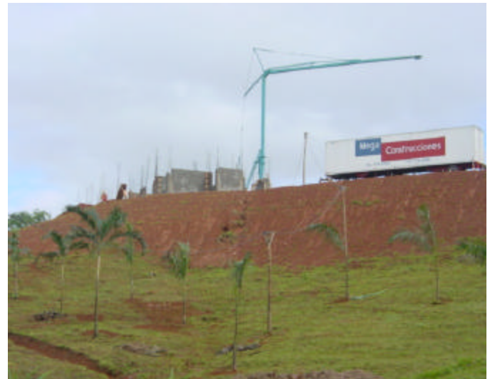
New roof lines on the horizon...
