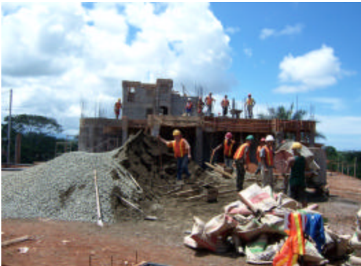
New Construction at Del Pacifico
