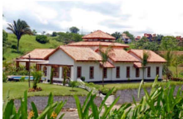
New house at Del Pacifico in the morning light.
